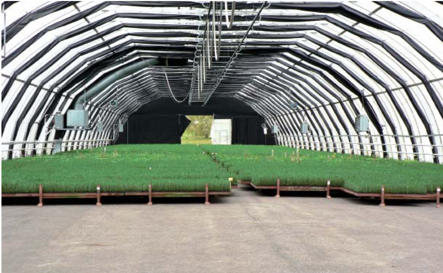
Greenhouse with heating and ventilation equipment and short-day treatment curtains (photo T. Saksa).
